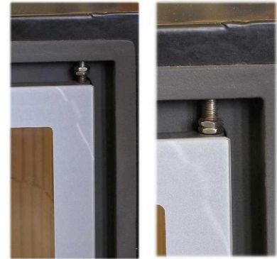
Illustration 28: Right: Nuts after mounting the door - Left: Door hinge after adjustment
